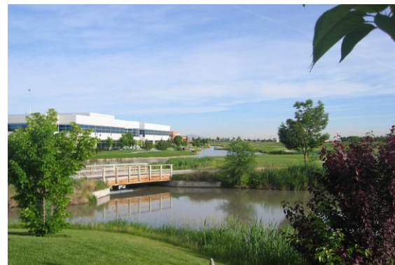
A pedestrian bridge spanning over one of the series of lakes - Phase I
